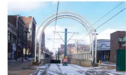
LIGHT RAIL PORTAL
