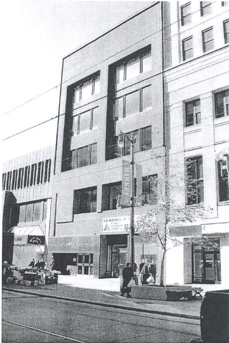
Photograph 50. East elevation of 410 Main Street, facing southwest (PCI 2001).
