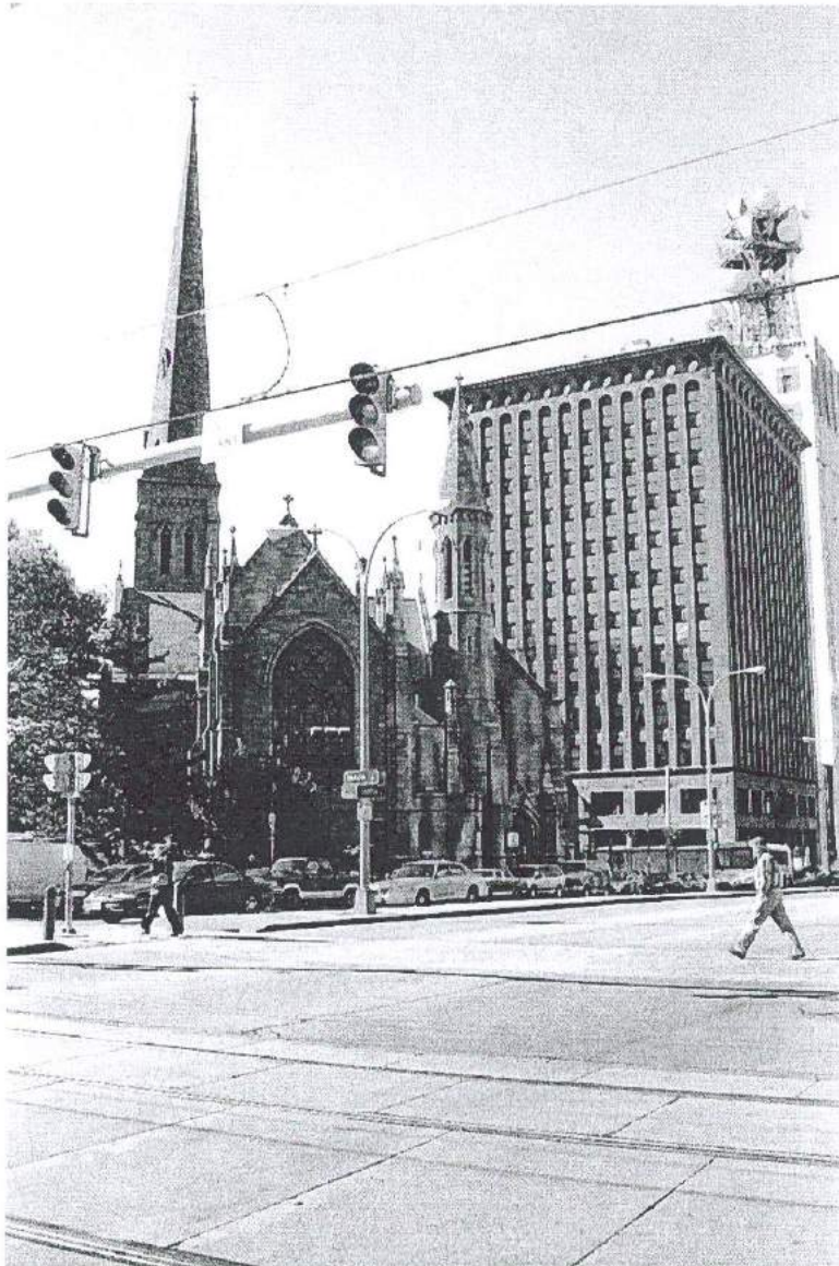
Photograph 9. Two National Register Listed buildings within the viewshed of the project area: St. Paul's Episcopal Cathedral Church, at left, and the Prudential Building, at right, facing southwest ( PCI 2001 ).
