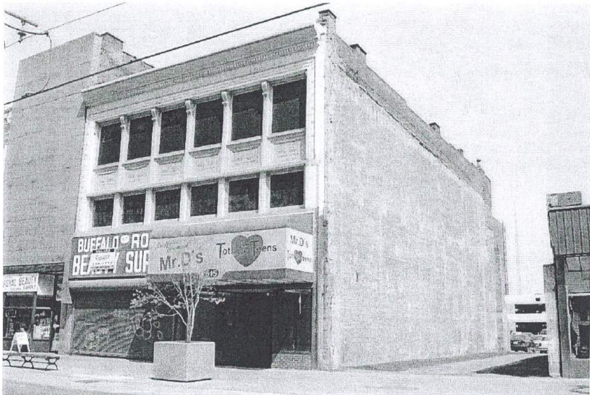
Photograph 66. West and south elevations of 515 Main Street, a contributing building of the NRE 500 Block Historic District. Note vacant lot at right, facing northeast (PCI 2001).
