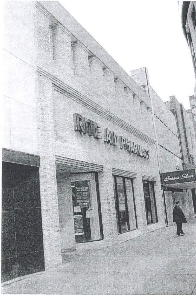
Photograph 55. East elevation of 450 Main Street, facing northwest (PCI 2001).
