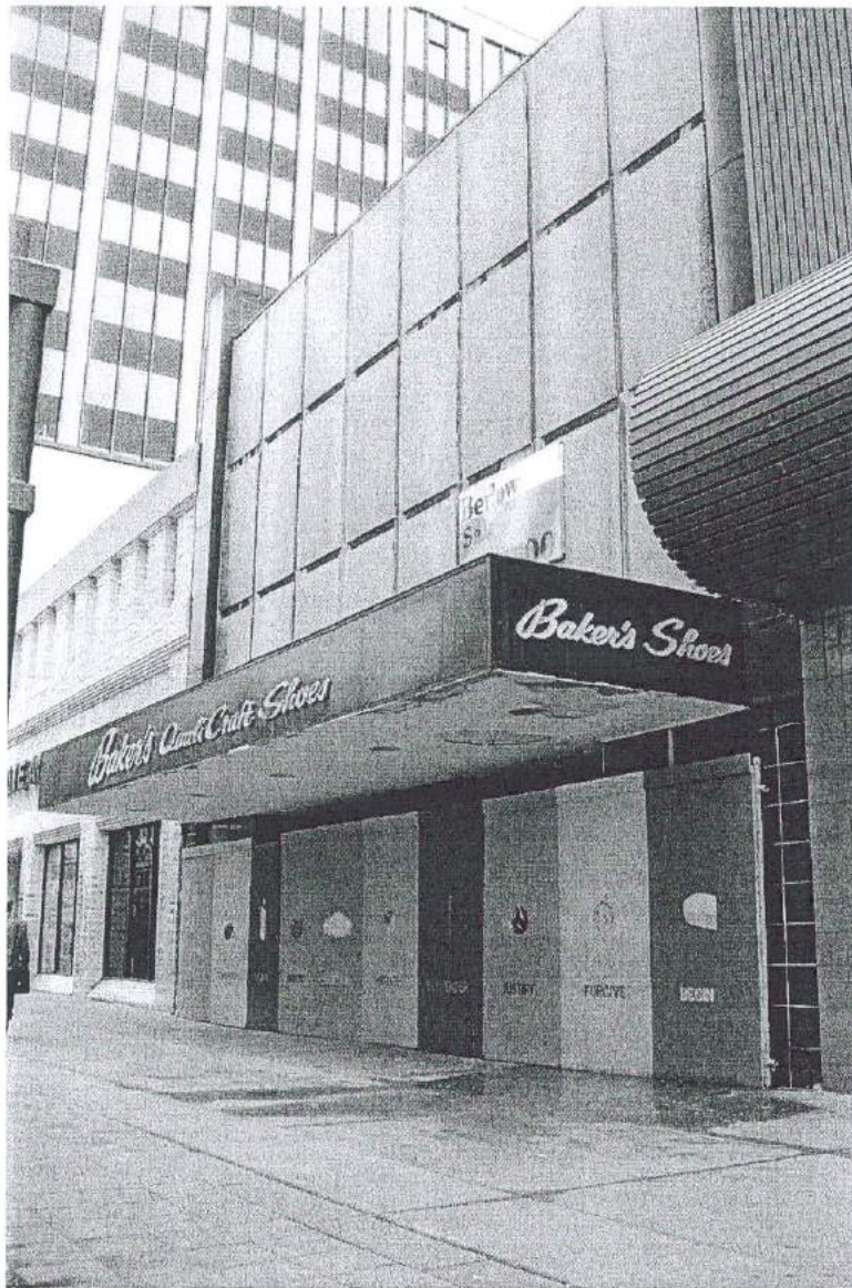
Photograph 56. East elevation of 456 Main Street, facing southwest (PCI 2001).
