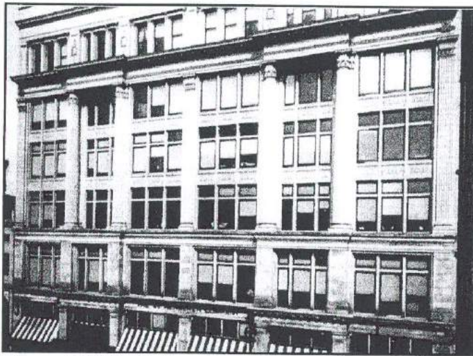
Figure 24. West elevation of the "new" Hengerer's department store as it appeared in 1903 (Western New York Heritage, 1998).
