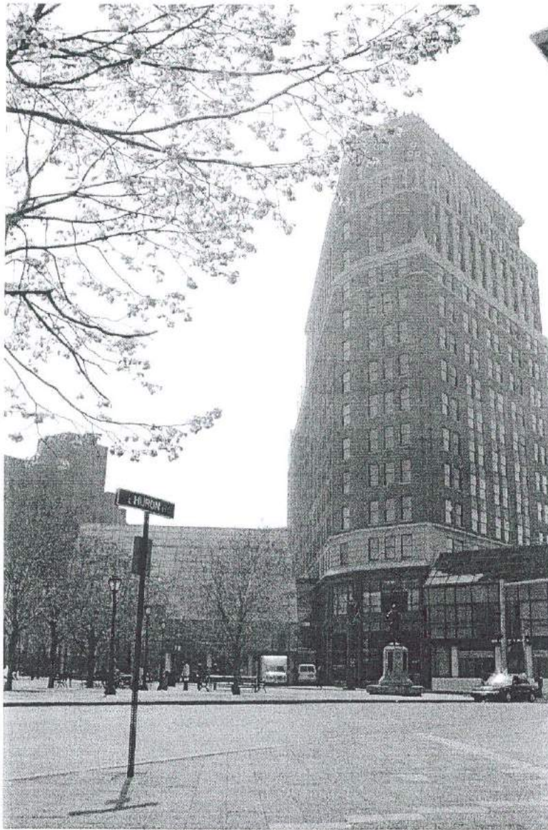
Photograph 76. Hyatt Regency Hotel at 2 Fountain Plaza (PCI 2001).
