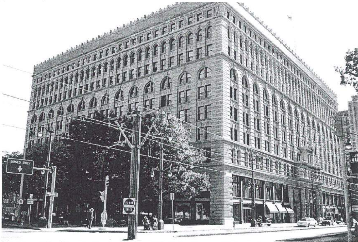
Photograph 40. North and west 295 Main Street (Ellicott Square Building), facing southeast. Note 295 Main Street is a contributing building of the Joseph Ellicott Historic District (PCI 2001).
