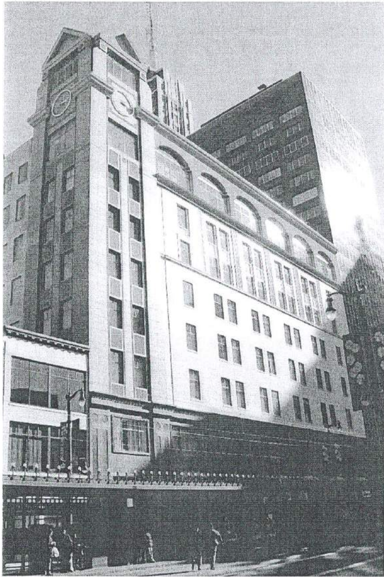
Photograph 58. West elevation of 465 Main Street, facing southeast (PCI 2001).
