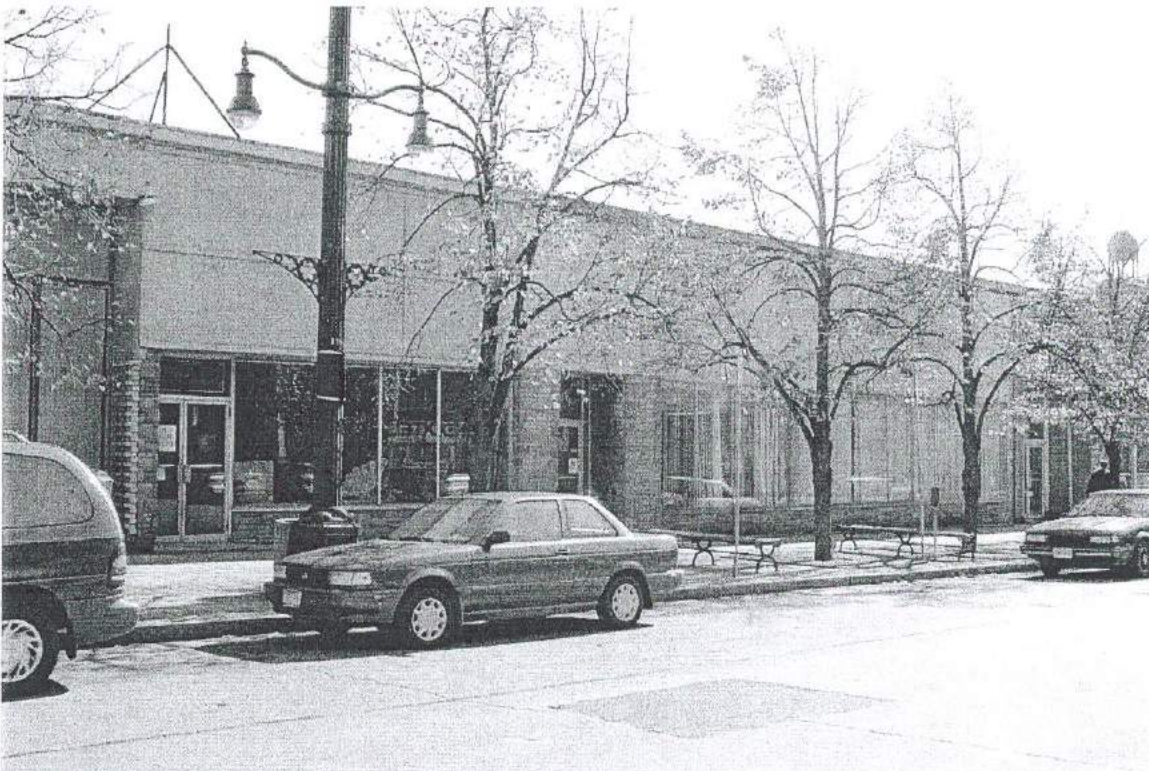
Photograph 109. 721 Main Street, facing southeast. Note 721 Main Street is a contributing building of the Theater District ( PCI 2001 ).
