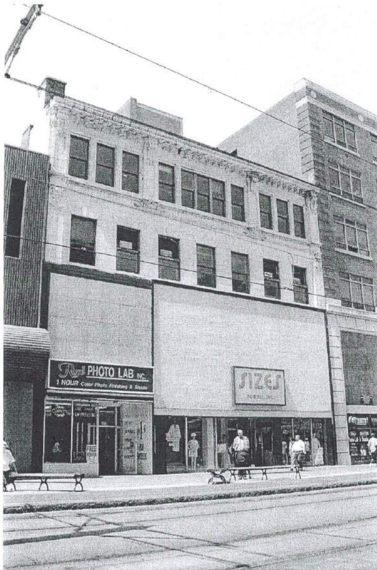
Photograph 59. East elevation of 472- 474 Main Street, facing northwest (PCI 2001).
