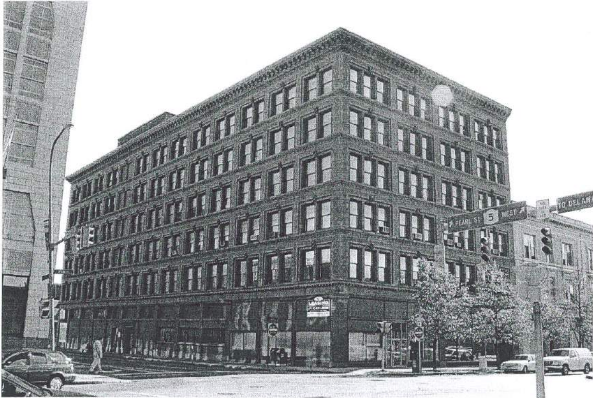
Photograph 120. 775-779 Main Street (Sidway Building), facing northeast. Note 775-779 Main Street is a contributing building of the Theater District ( PCI 2001 ).
