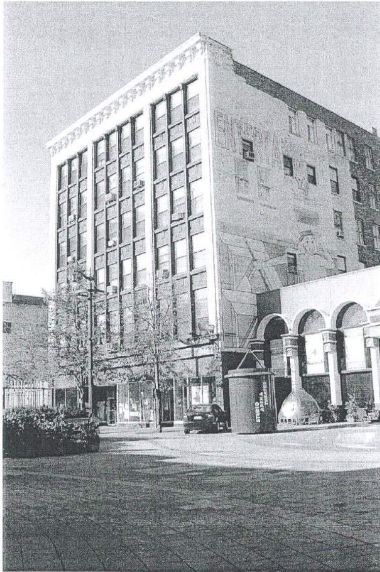
Photograph 103. 698-702 Main Street (Byer Building). Note 698-702 Main Street is a contributing building of the Theater Historic District (PCI 2001).
