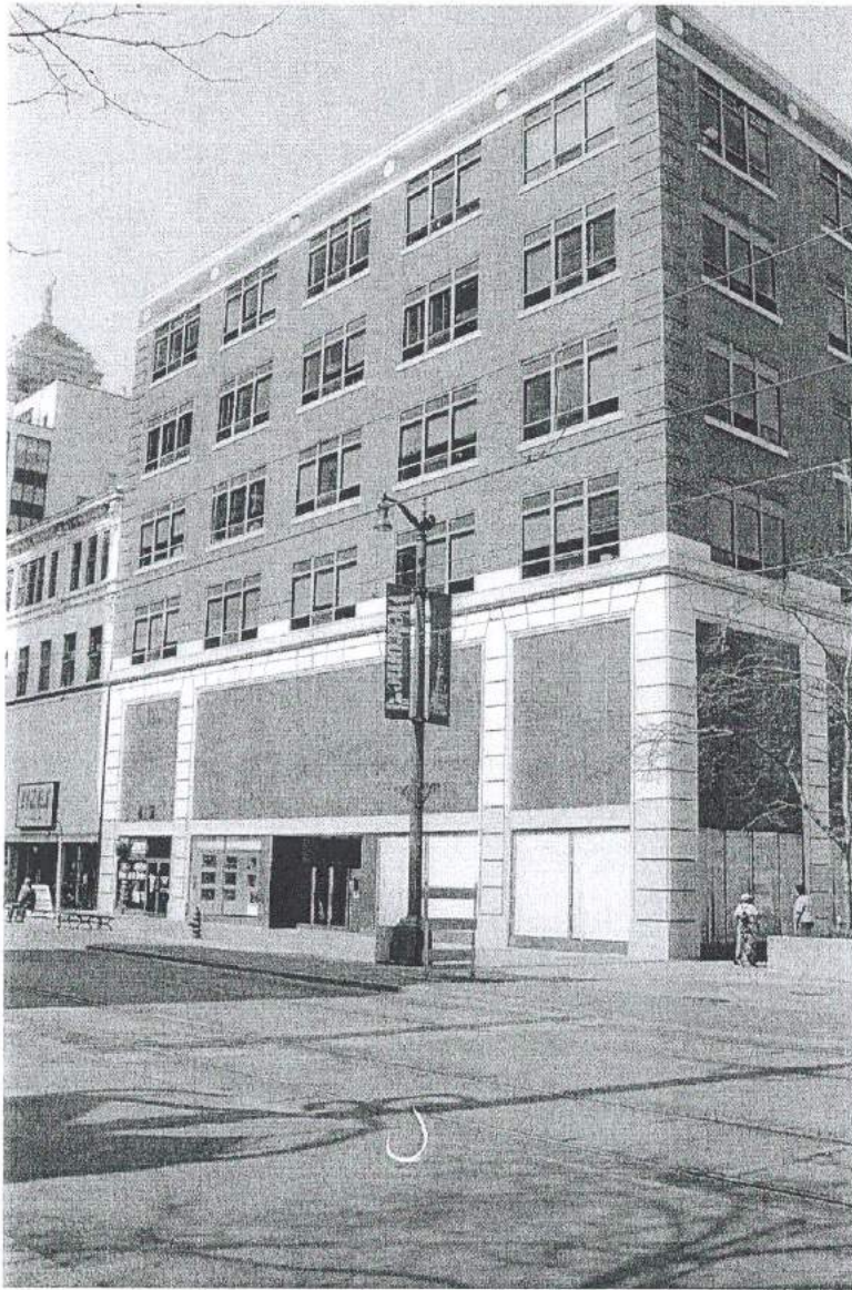
Photograph 60. East elevation of 478 Main Street, facing southwest ( PCI 2001 ).
