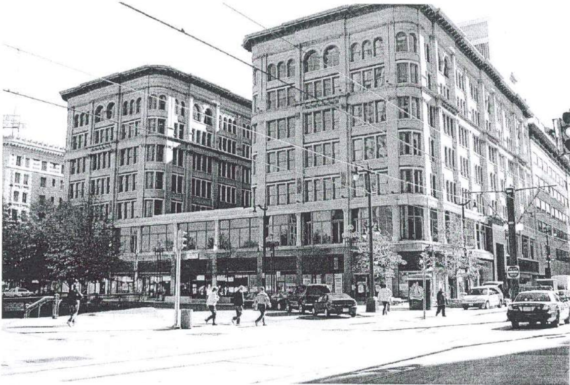
Photograph 49. North and west elevations of 395-403 Main Street (Brisbane Building), facing southeast. Note 395-403 Main Street is individually eligible for listing in the NRHP and occupies the south side of Lafayette Square (PCI 2001).
