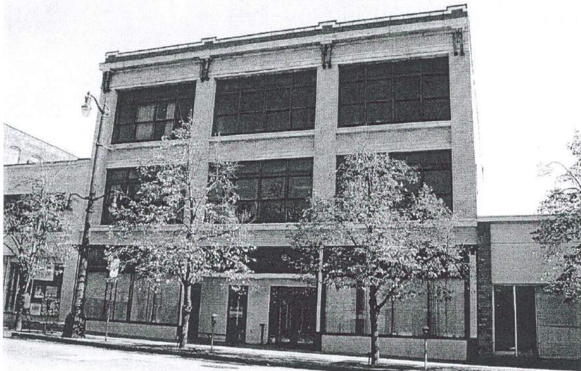
Photograph 111. 733-737 Main Street, facing east-northeast. Note 733-737 Main Street is a contributing building of the Theater District ( PCI 2001 ).
