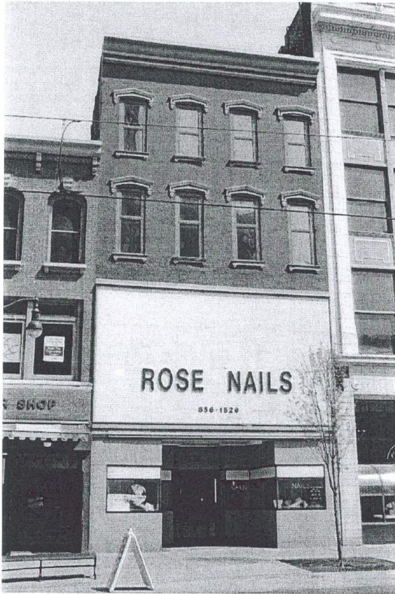
Photograph 70. West elevations of 535 Main Street, a contributing building of the NRE 500 Block Historic District, facing east (PCI 2001).
