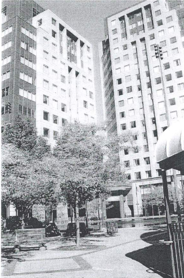
Photograph 79. One Fountain Plaza (Key Center and Rotary Rink), facing northwest. Note the south tower is at left and the north tower is at right ( PCI 2001 ).
