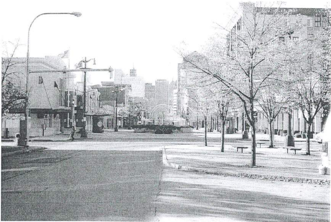
Photograph 24. Main Street with the northern end of the LRRT tunnel in center, facing south (PCI 2001).
