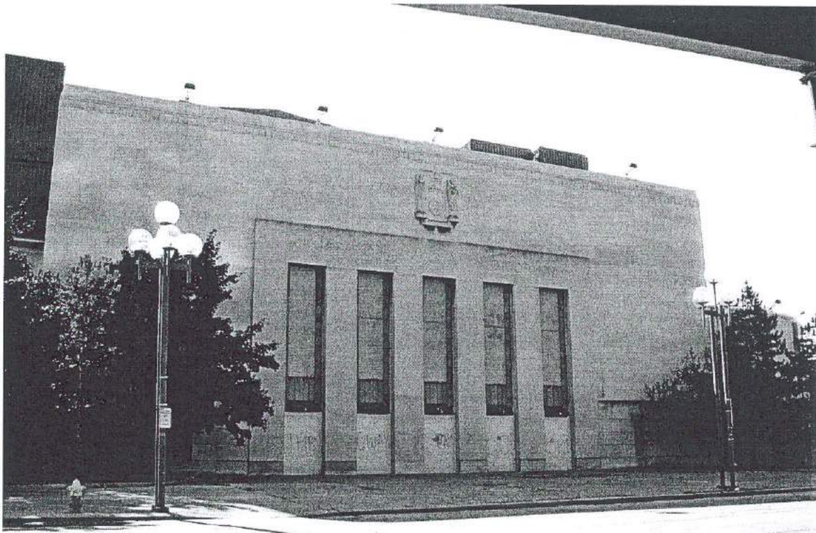
Photograph 30. North elevation of Buffalo War Memorial Auditorium (130 Main Street), facing south (PCI 2001).
