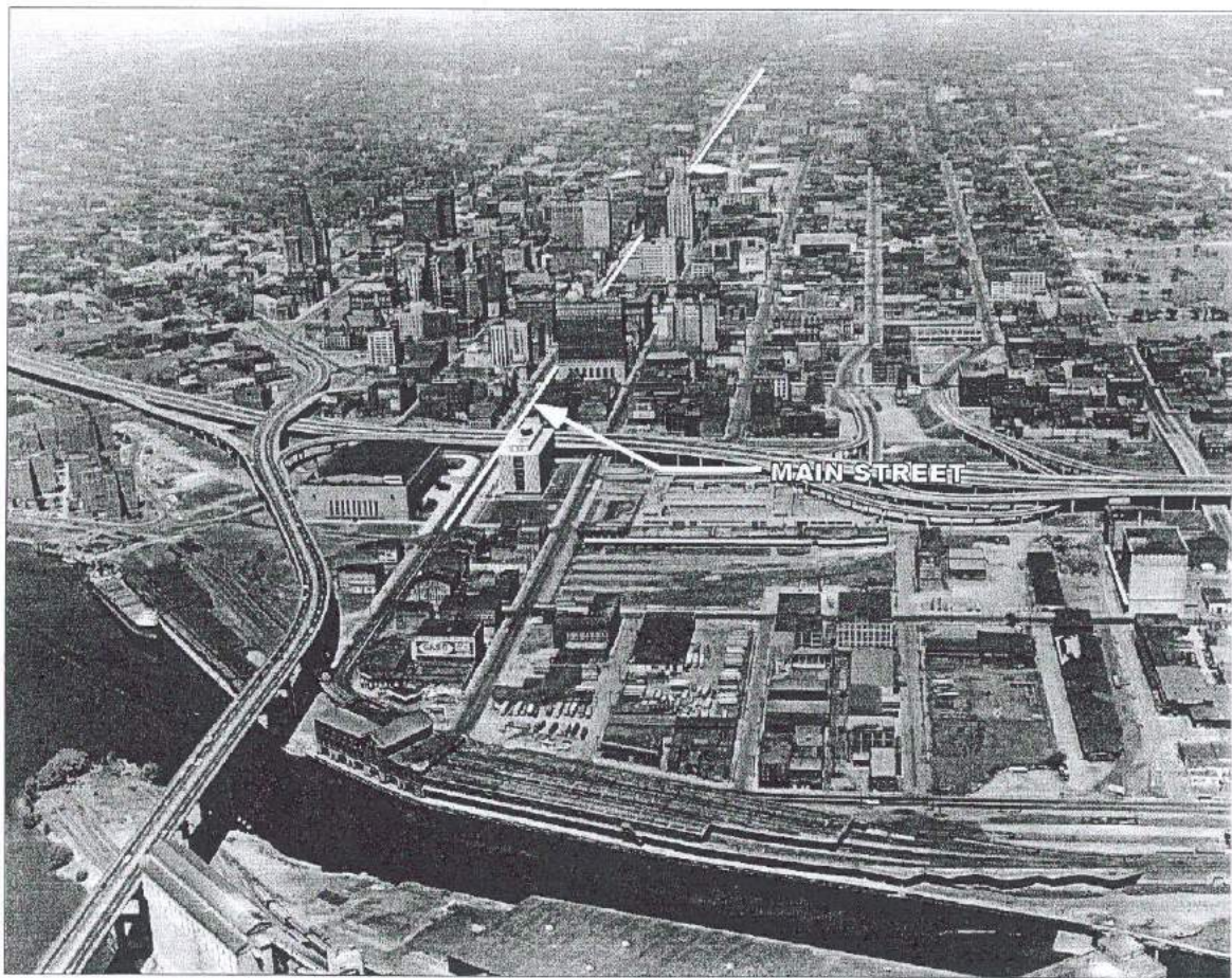
Figure 14. The Main Street project area after completion of the I-190, ca. 1964 (Leary and Scholes 1997).
