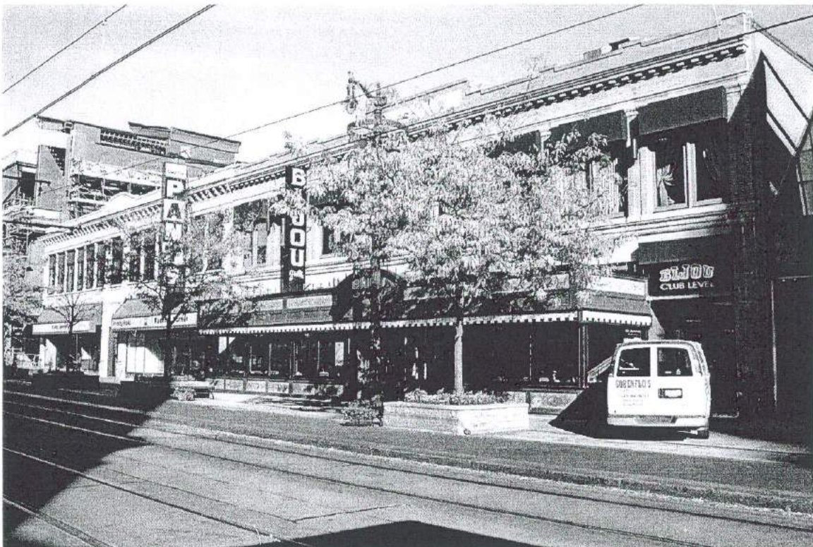
Photograph 91. 643-649 Main Street (Dold Building), facing northeast. Note 643-649 Main Street is a contributing building of the Theater Historic District (PCI 2001).
