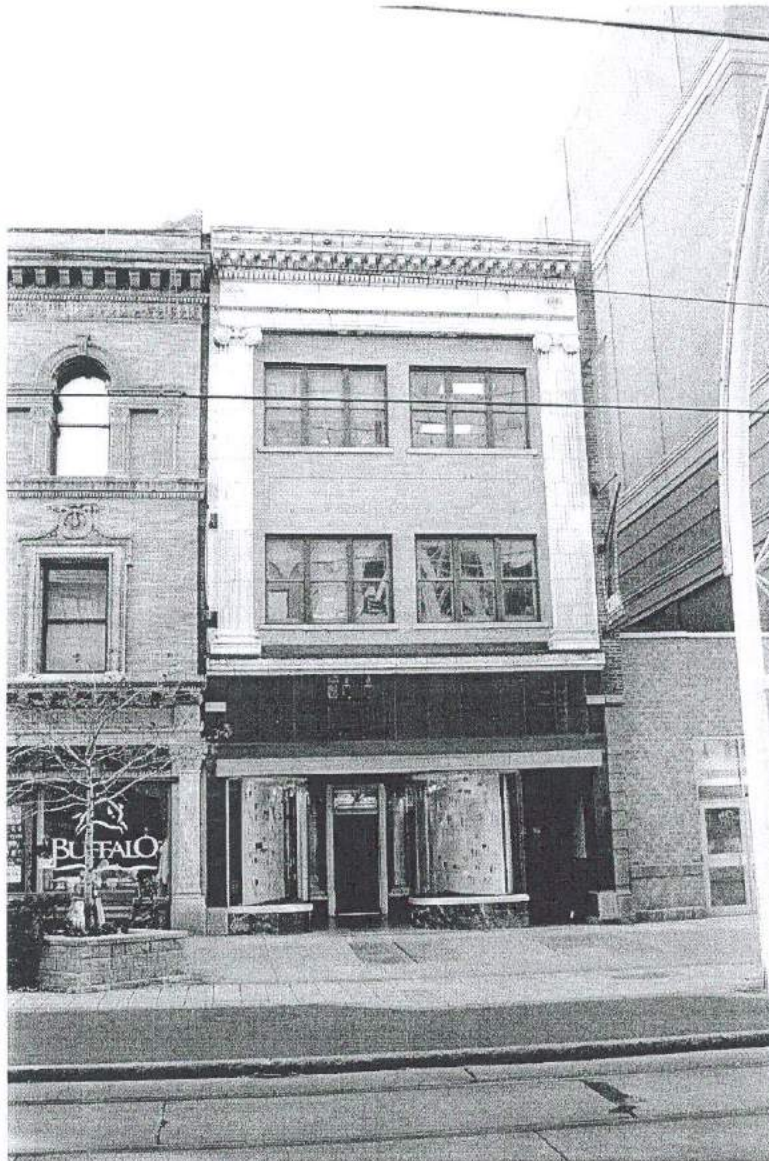
Photograph 82. West elevation of 615 Main Street (CEPA Gallery), facing east. Note 615 Main Street is a contributing building of the Theater Historic District (PCI 2001).
