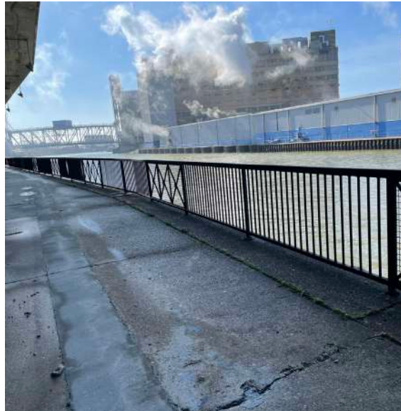
CONCRETE TRAIL SURFACE CONDITION
