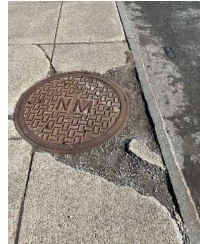
SIDEWALK CRACKING
