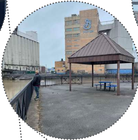
Approximately 5,000 sf of an asphalt area with a pavilion is located near the eastern edge of the study area along the trail.
