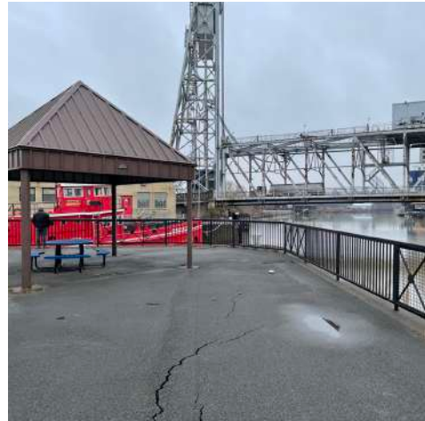
EXISTING PAVILION AREA
