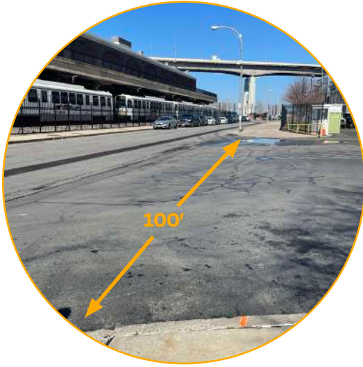
1 The KeyBank Center and parking garage driveway presents a 100' gap in the pedestrian right-of-way.
