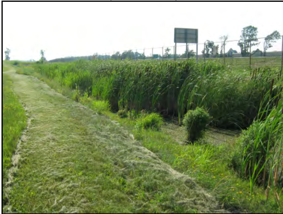
Photograph 7: Drainage channel outside of the NYS Thruway eastbound right-of-way fence. Channel is along the north edge of the wetland on the Runway 23 end, but is divided by the mowed berm pictured along the left side of this photograph. (MJ Photo 07/06/10)
