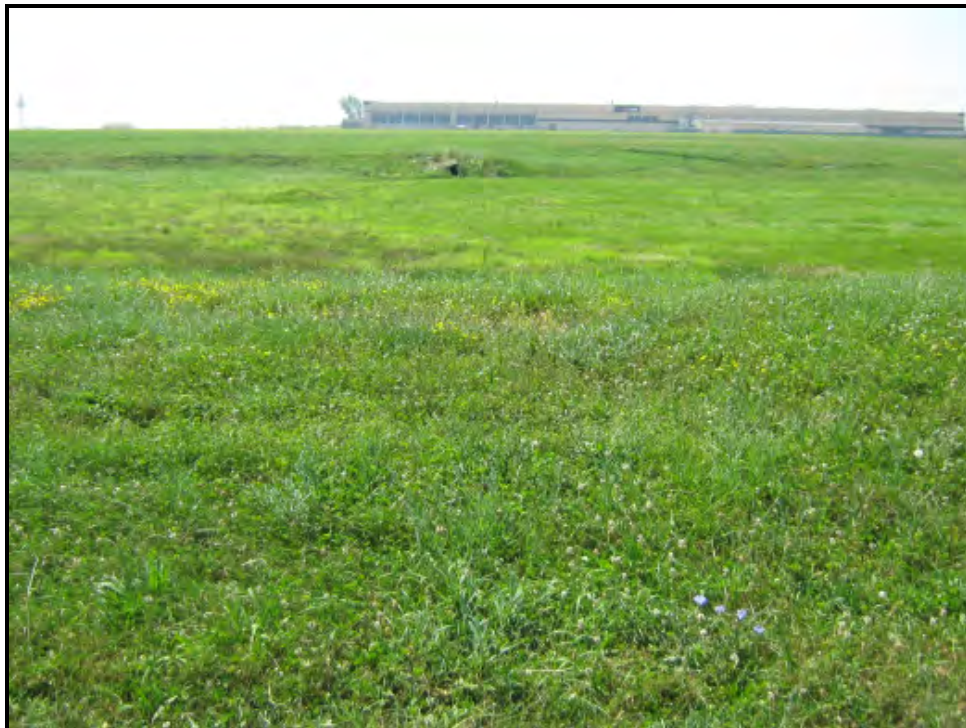
Photograph 10: Retention Basin "A" at the Runway 14 end near Werle Drive looking to the south from the perimeter road. The area is a rectangular basin identified as wetland in the previous study. (MJ Photo 07/07/10)
