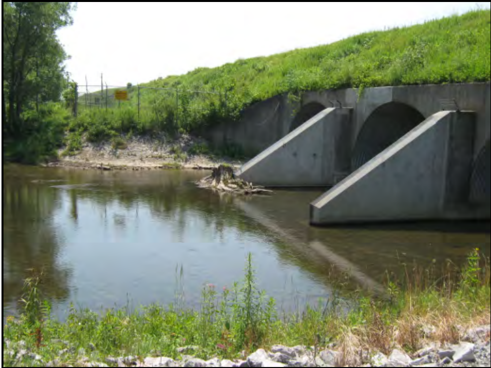
Photograph 17: Ellicott Creek upstream of Runway 23 culvert. (MJ Photo 07/07/10)
