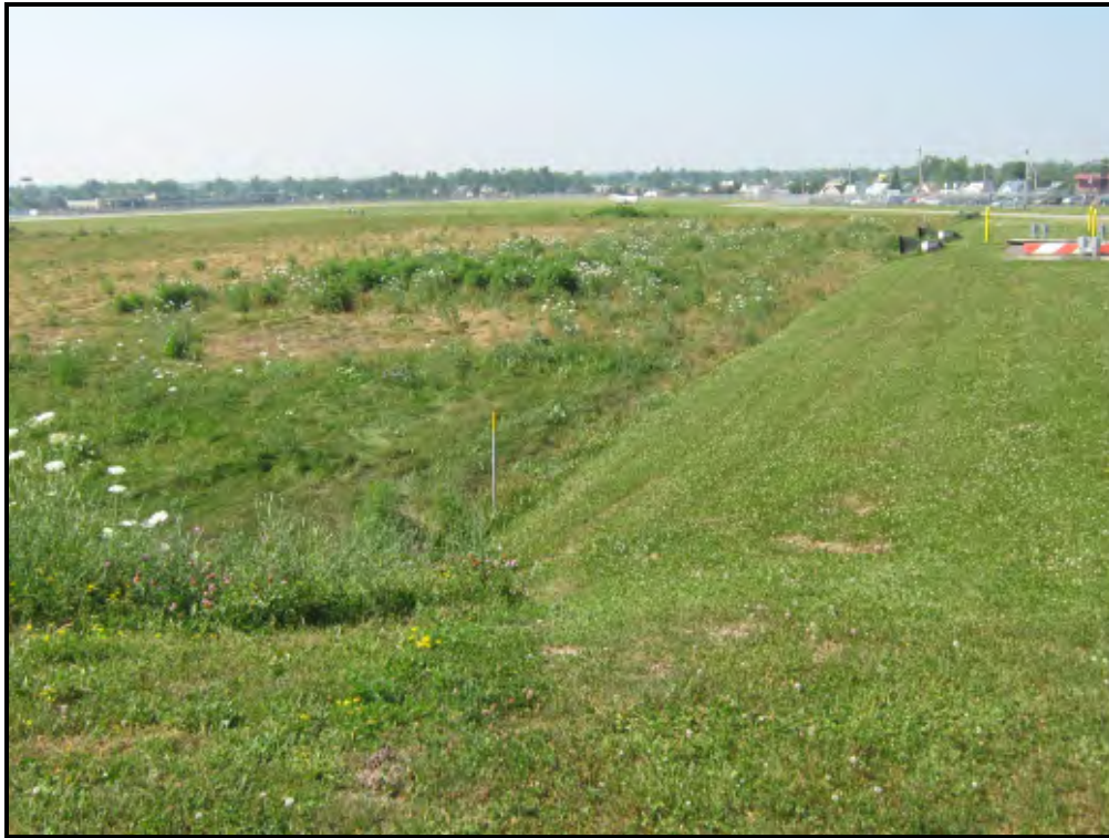
Photograph 11: BNIA's engineered underground wetland for glycol treatment. This photograph shows the #4 cell looking towards the west. (MJ Photo 07/07/10)
