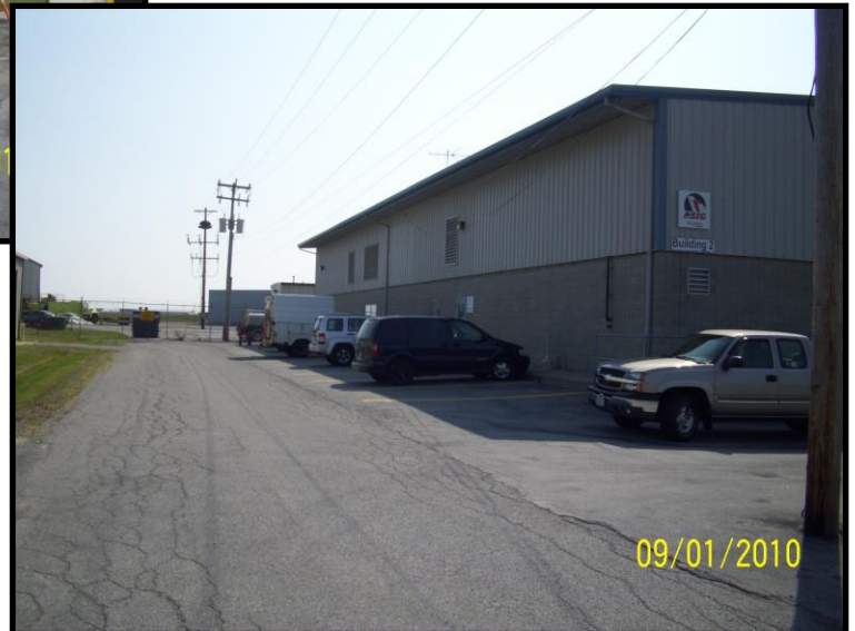
Ground Support Equipment Building – North Side
