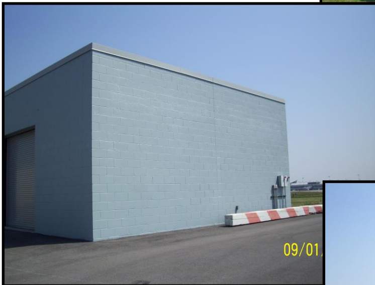
Glycol Treatment Utility Building – Northwest Side
