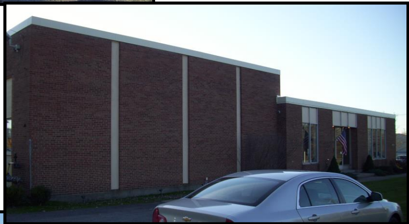
235 Aero Drive – North Side
