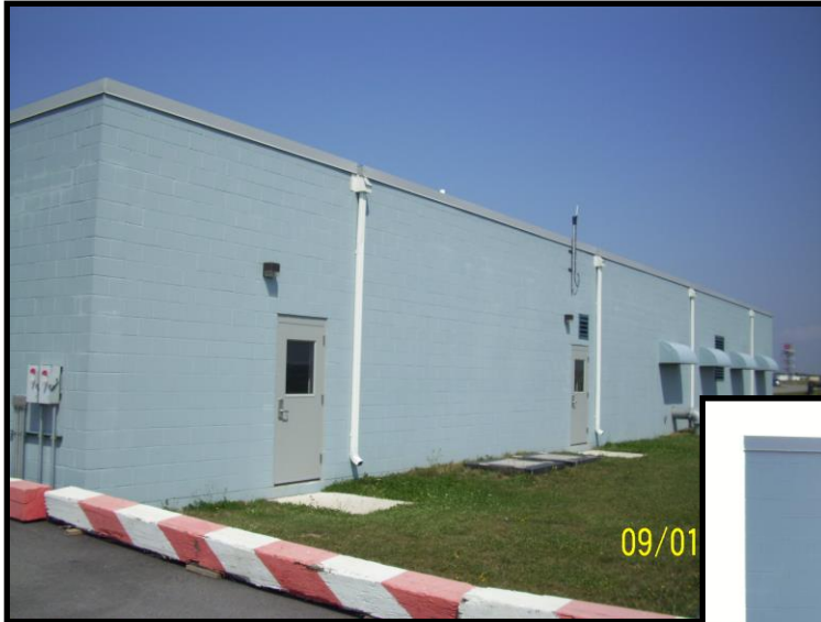
Glycol Treatment Utility Building – Northeast Side
