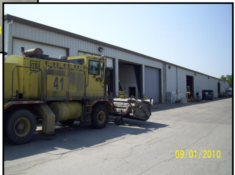
Maintenance Garage – East Side
