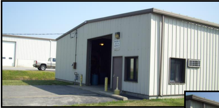
Maintenance Building – West Side
