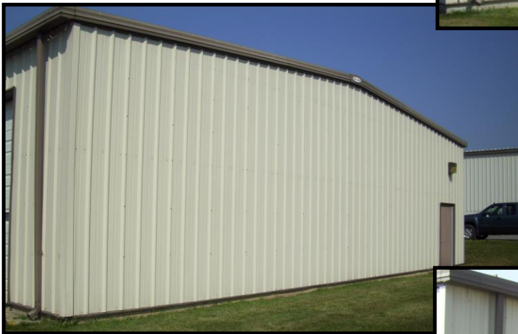
Maintenance Building – East Side
